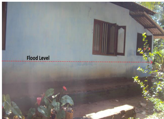
Figure 8: Raising of doors and windows
